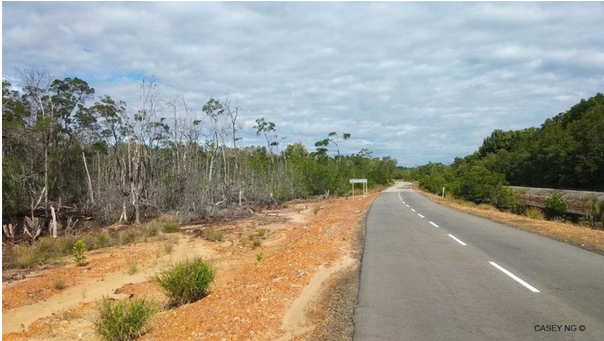
Figure 5. An example of coastal road development that disturbed the natural intertidal hydrology and caused mangroves to die-off. Such a problem would have been easily resolved if the road was engineered with more culverts that enable free flowing of tidal waters.
